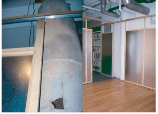
Rhona Hoffman Gallery partitons, Corpopolis/OSB Design/Build, Chicago 1996 Sliding partitions fabricated from off the shelf wooden brick moulding and sheets of galvanized sheet metal. Corpopolis/OSB was an after work collective of DHoffman, JKaufman, RKober, BNorsman. We maintained a shop, dsesigned, and built several collective projects for 3 years.
