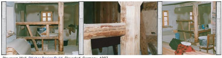
Playroom Wall, RKober Design/Build, Gleusdorf, Germany, 1987 Itinerant Timber Framer Apprentice Piece. The room divider is made of repurposed timbers. The column is from a 19th century industrial building. The partition members are from barn rafters. All connections are hand-made mortise and tenon.
